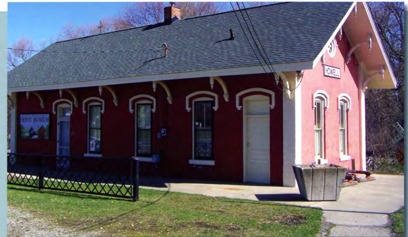
The Ann Arbor Railroad Depot was built in 1886, fifteen years after the first train stopped in Howell. Today, it serves Howell as a museum.
